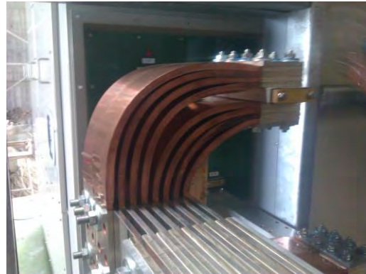
DC Device lead to Terminal
