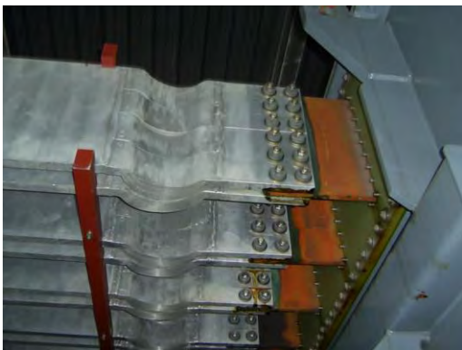
Movable parts of switch
