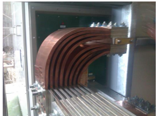
DC Device lead to Terminal
